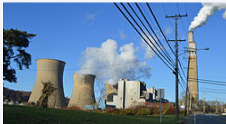
Bruce Mansfield plant
