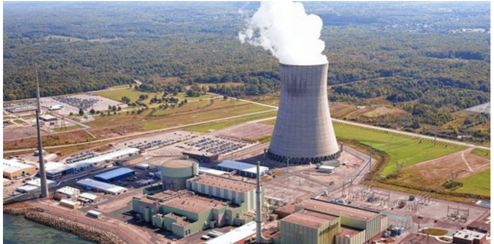
Nine Mile Point Nuclear Plant | Constellation Energy Nuclear Group
