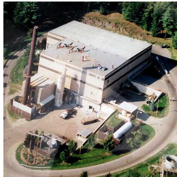
Claremont energy-from-waste facility | Stuart B. Millner & Associates
