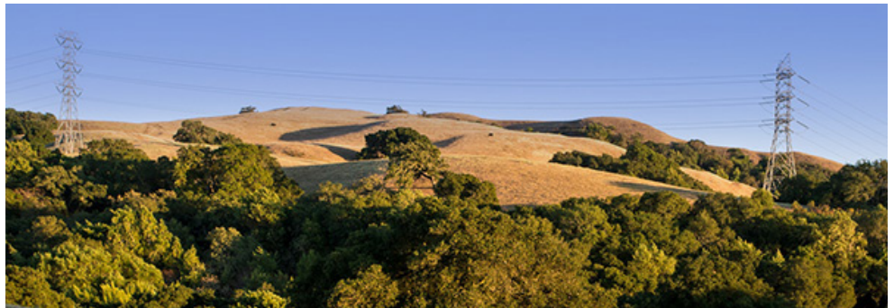
Power lines in Contra Costa County, California | USDA
